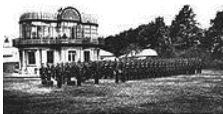
Ordnance Survey Photography Building
